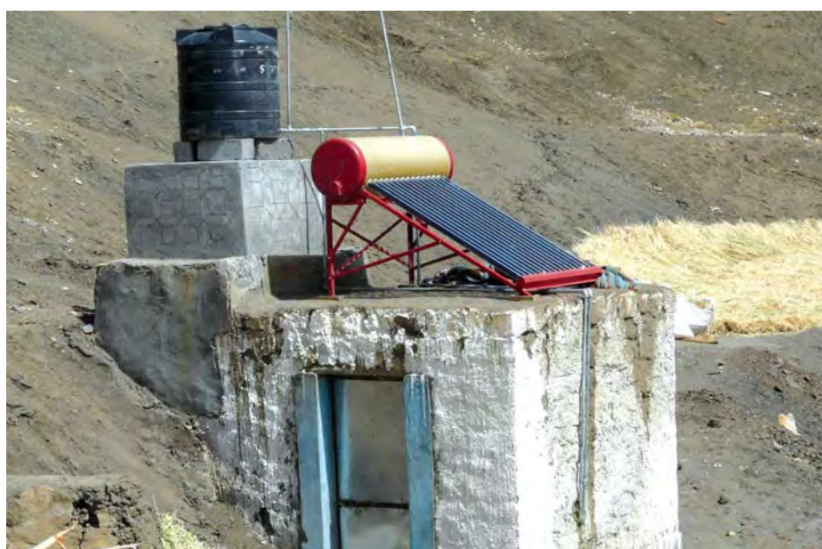
Solar water heater on the common bathing facility introduced by Muse to improve tourism facilities in the project villages
