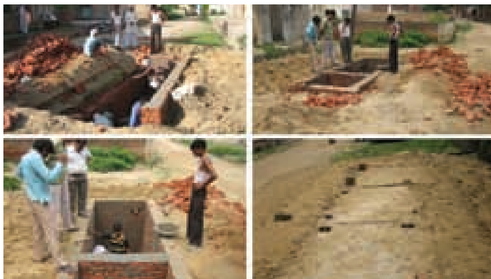
Intallation of traditional sewage treatment system at Karnabas village
